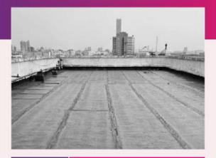
**Objective:** The primary objective of the Commerce House project was to implement a robust roof waterproofing solution using an APP membrane, complemented by screed concrete to ensure long-term protection of the membrane from potential damage. The project was planned for a duration of two months starting from May 2024.
